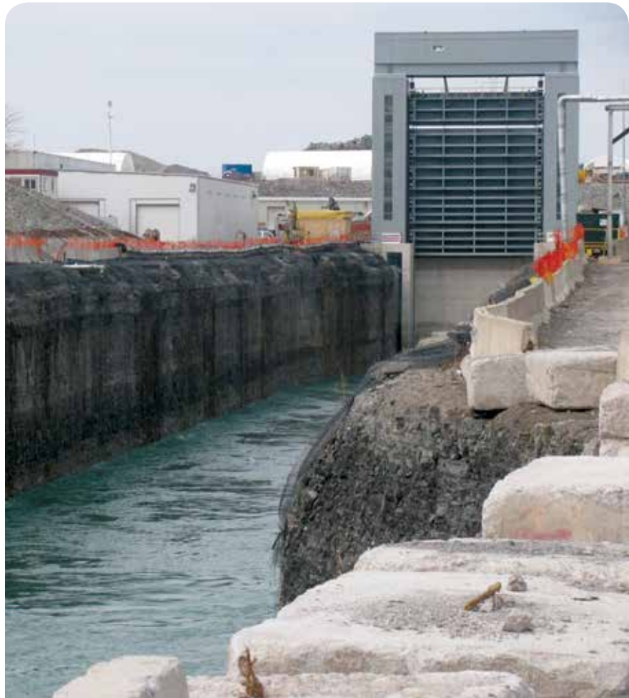
New Niagara Tunnel outlet tunnel and gate
