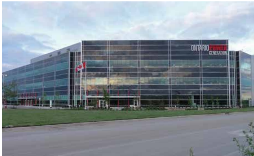
Darlington Energy Complex located in Courtice, Ontario.
