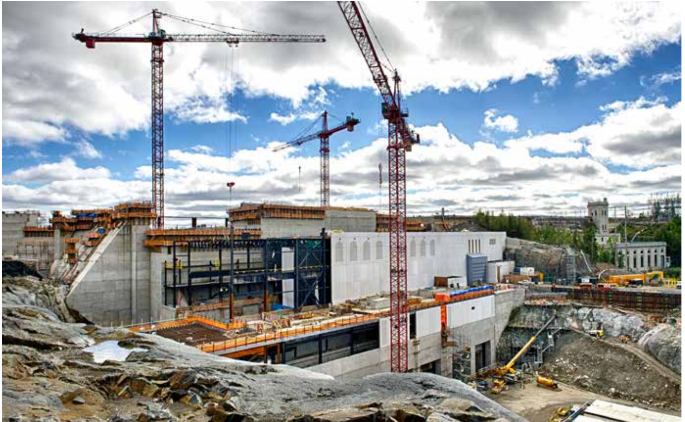
Construction at the Smoky Falls Generating Station
