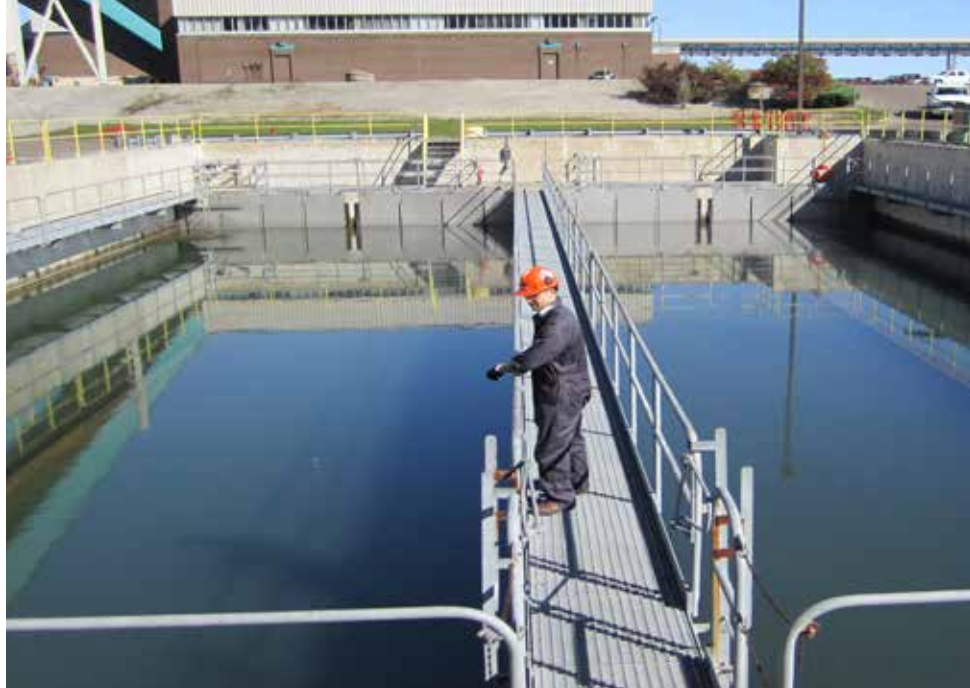
Inspection of an oily water separator at Nanticoke Generating Station
